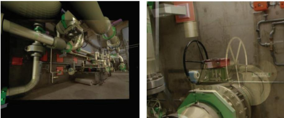
**Figure 1.12** AR can be used for discrepancy analysis in industrial facilities. These images show still frames overlaid with CAD information. Note how the valve on the right-hand side was mounted on the left side rather than on the right side as in the model. Courtesy of Nassir Navab.
